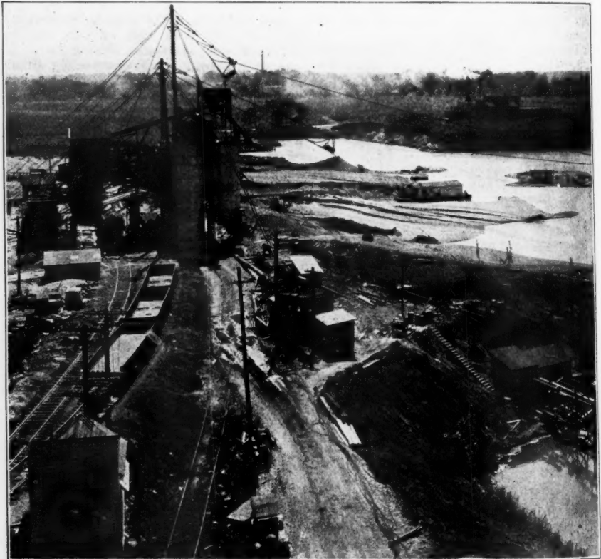
The Two-Unit Plant at Indianapolis
